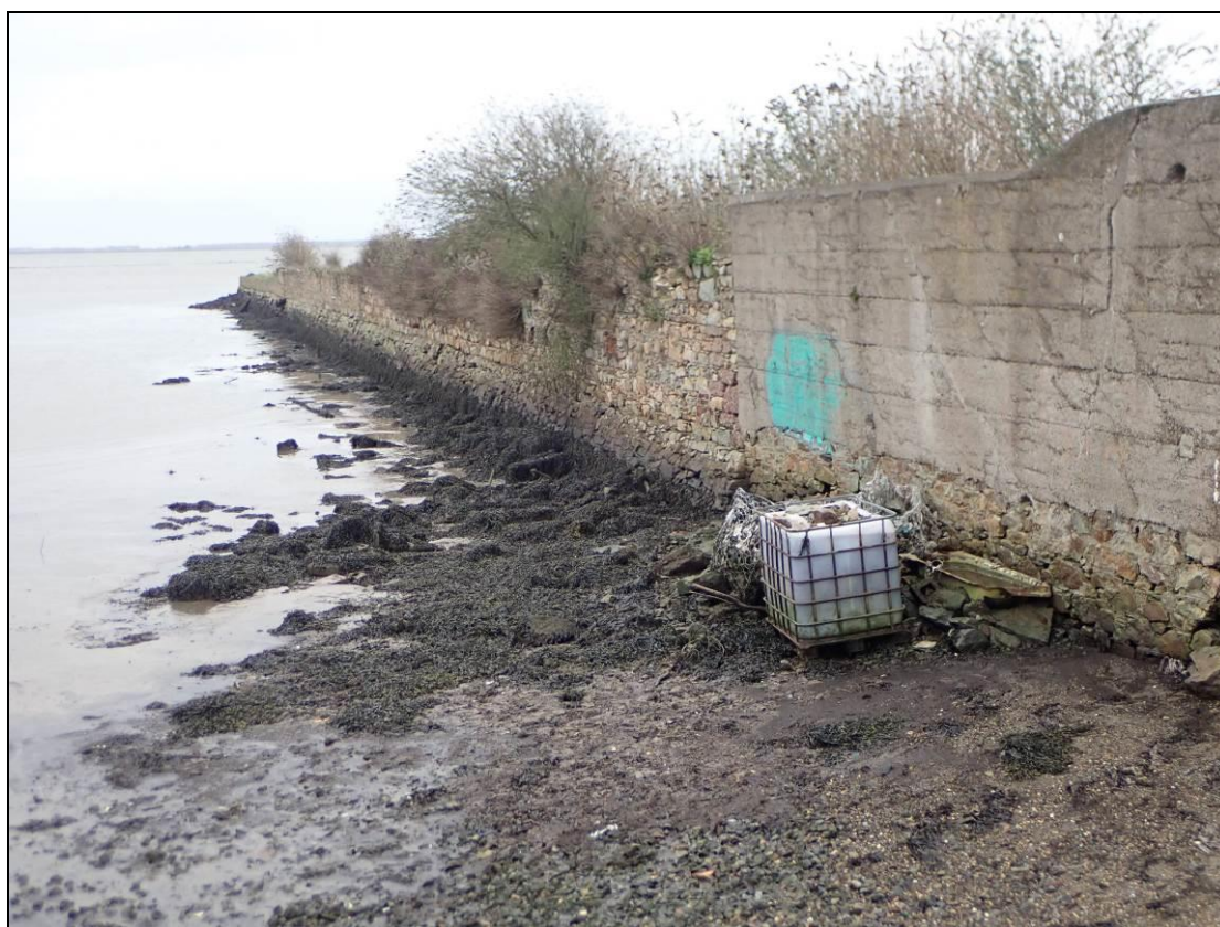
Plate 2: North-facing boundary wall of Trinity Wharf, that served originally to define the edge of the nineteenth-century dockyard. The concrete additions are later.
