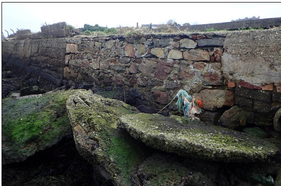
Plate 4: View looking west at river-frontage of Trinity Wharf. The stonework relates to former elements of the dockyard while the later concrete additions either side may mark where infill of the patent and related slipways has taken place.
