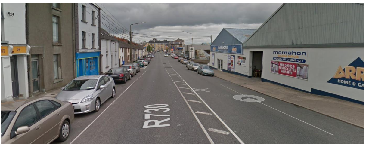
Figure 5- Trinity Street View in direction of Town Centre (North) from Proposed Access – one lane in each direction with on-street parking on both sides and ghost central median
