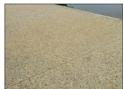
Proposed Exposed Aggregate Paving
