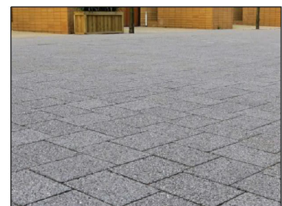
Proposed Concrete Paving Blocks
