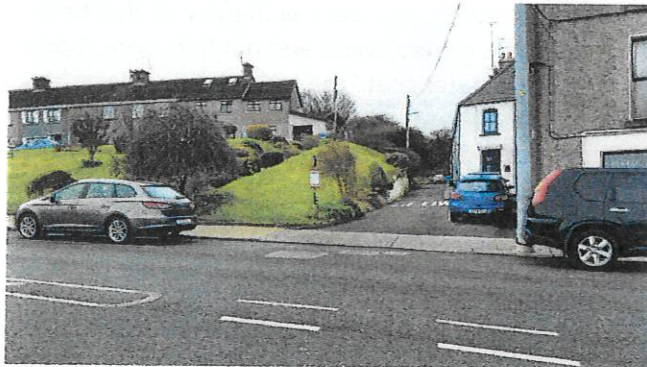
Image 4 Current access/ exit from Seaview Avenue. Note the sightlines available to drivers exiting the avenue to the footpath and from pedestrians into the Avenue. The proposed junction redesign would remove sightlines for pedestrians and drivers from/to the south of the junction.
