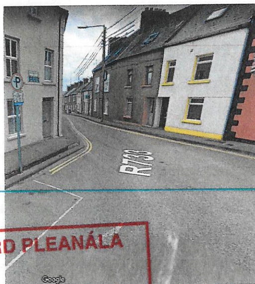
Image 10: Kevin Barry Street – junction at The Swan in The Faythe [Source: Google Streetview]
