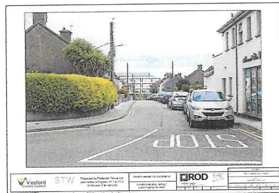
Image 26: View from Fisher's Row/The Faythe Junction
