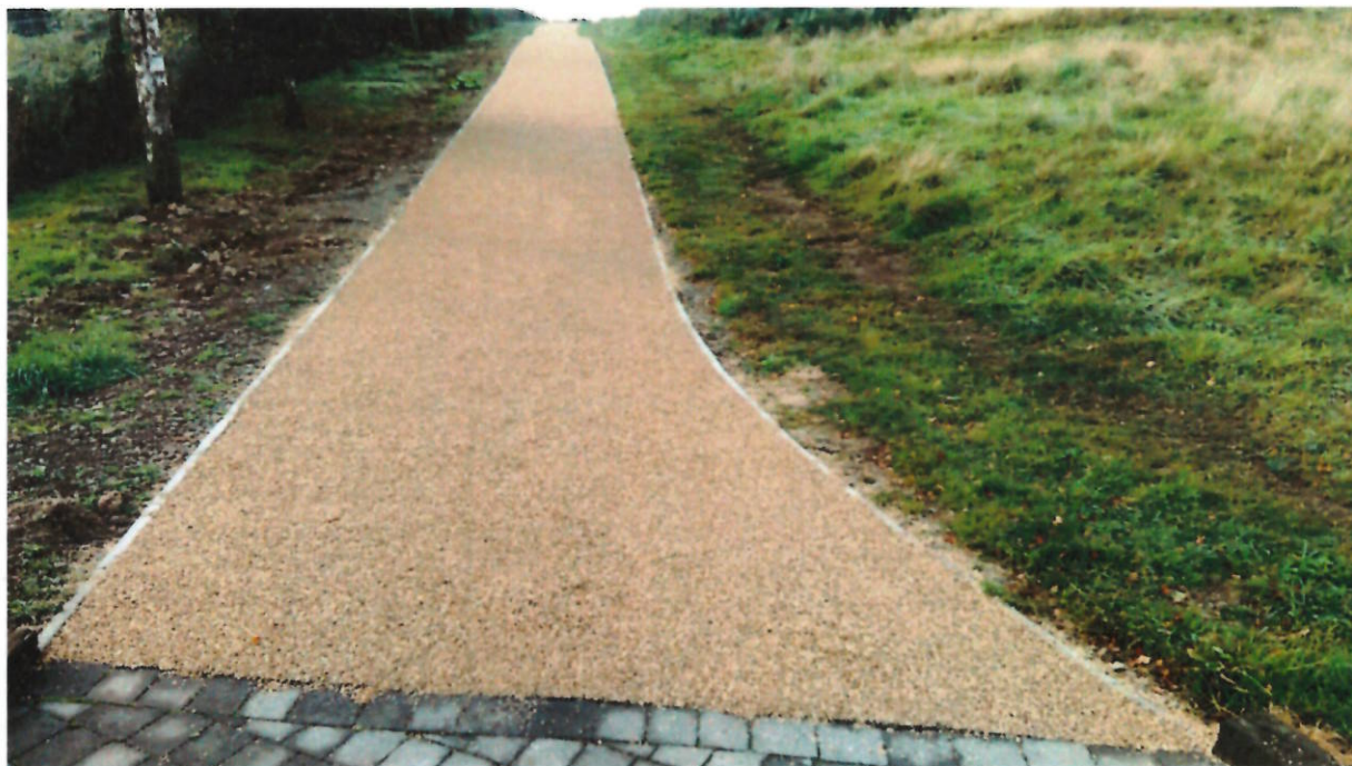
TCD / 1000 /01: Resin Bound Granular Surface:
