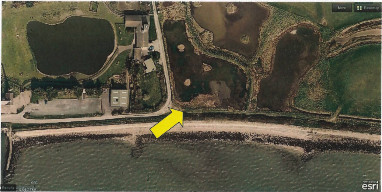
Fig. D1: Winter Close Section at Location No.1.
