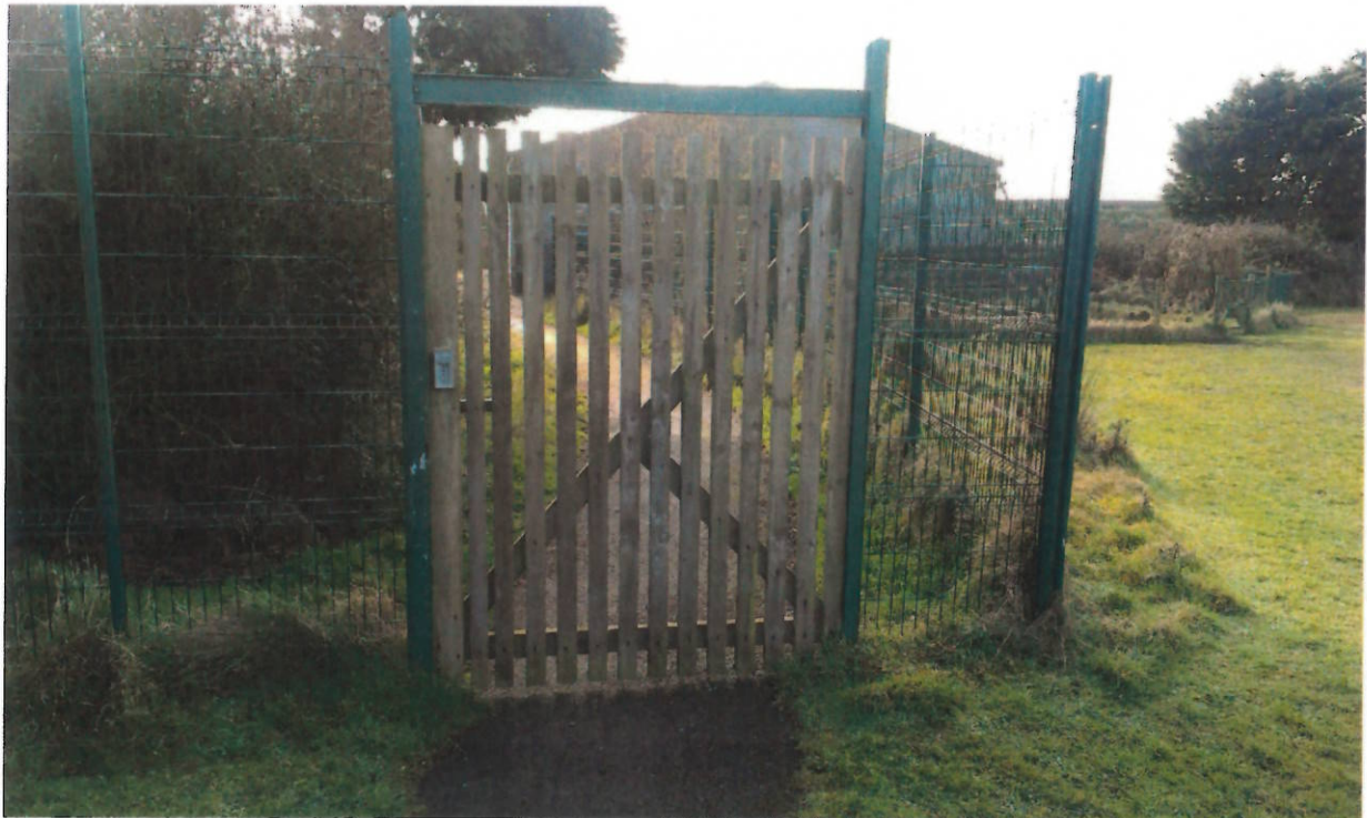
Fig. D5: 2.4m High Paladine Fencing, close spacing of grid makes climbing impossible.
