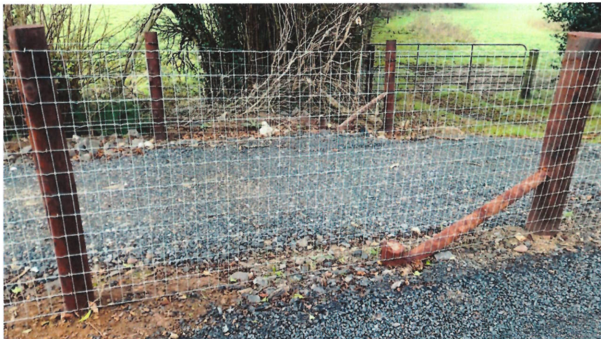
TCD / 300 /01: Timber Post & Narrow Ope Sheepwire Fence: (kerb required at fence base to contain dogs on the trail)
