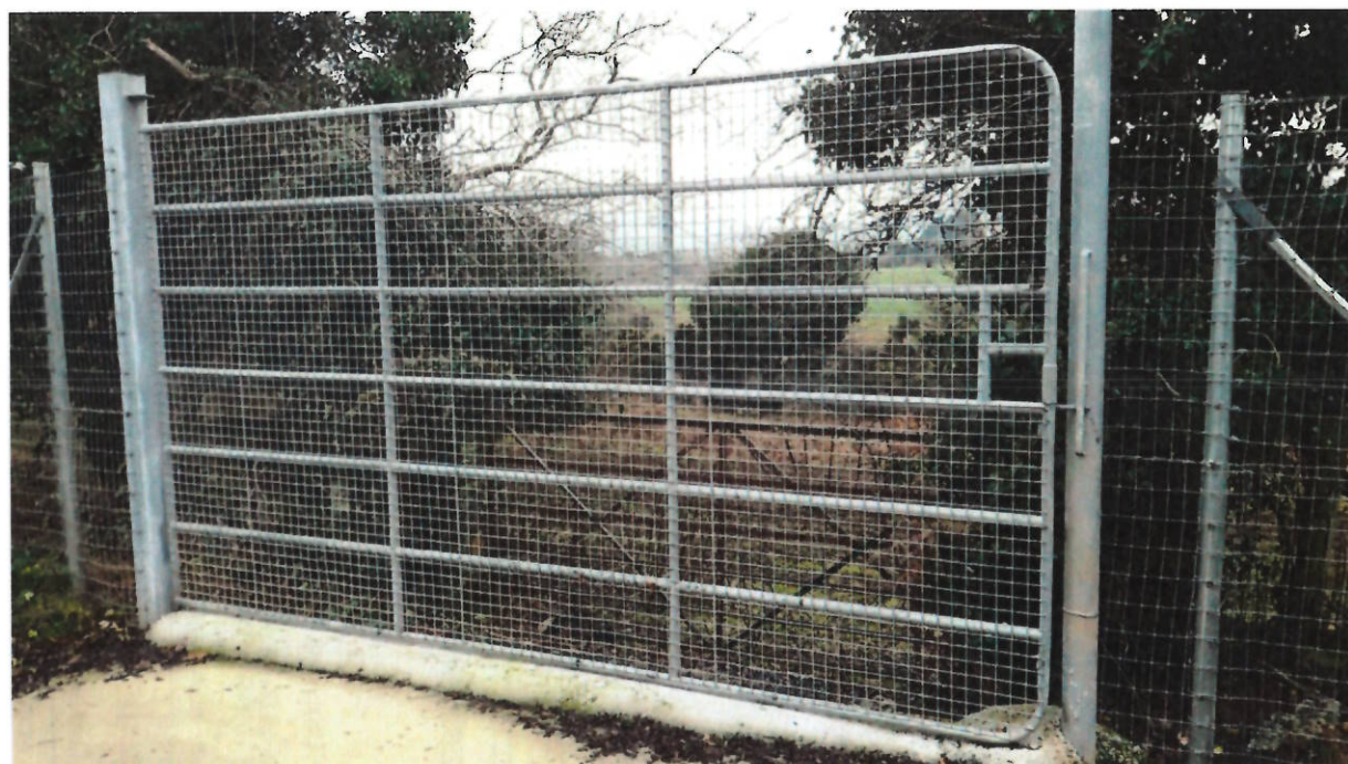
TCD / 300 /09: Steel Single Field Gate (with square mesh):
