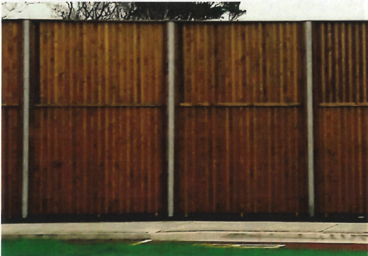
Fig. 5: Timber Clad Screen (2.4m High !).
