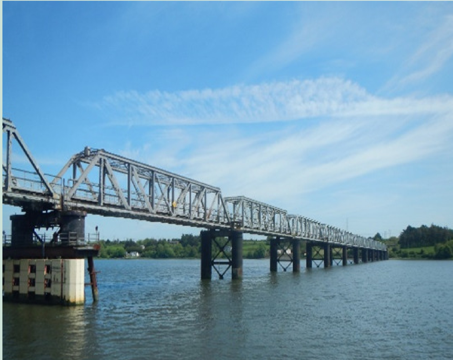
Barrow Bridge (approx 670m long 15 span bridge)
