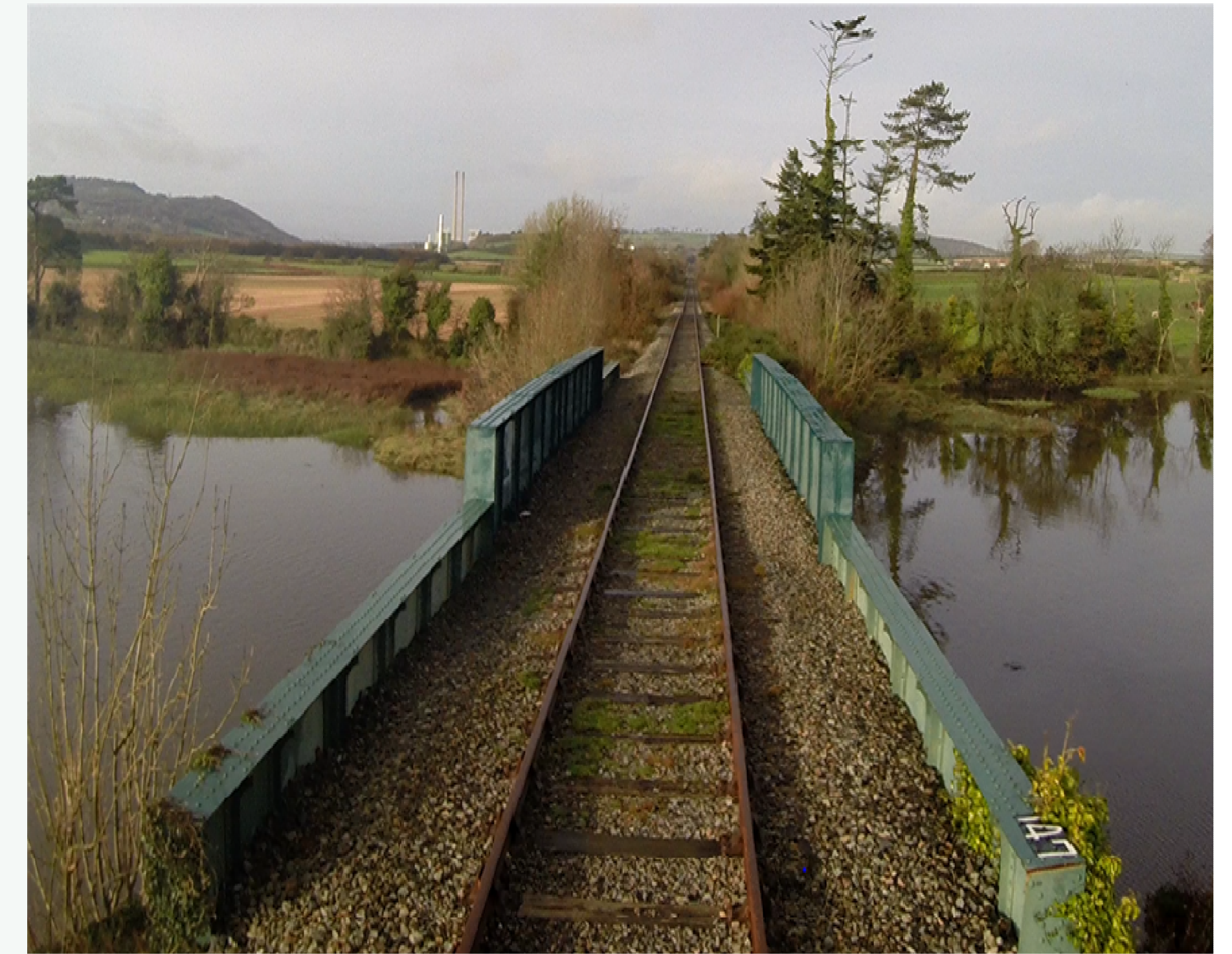
Campile River Bridge (approx. 35m long, 3 span bridge)
