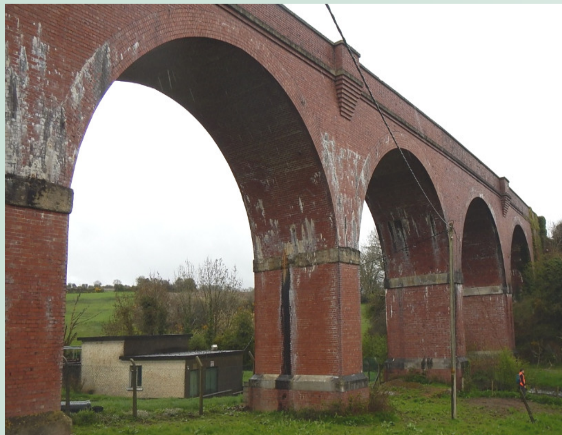
Taylorstown Viaduct (bridge deck approx. 5m wide)
