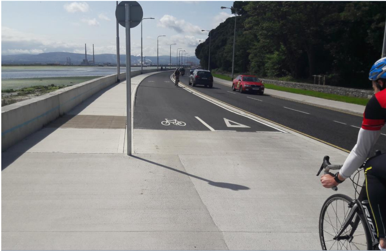
Fig. 6.2: Dual Cycle Lanes Applied to Clontarf Road, Dublin:
