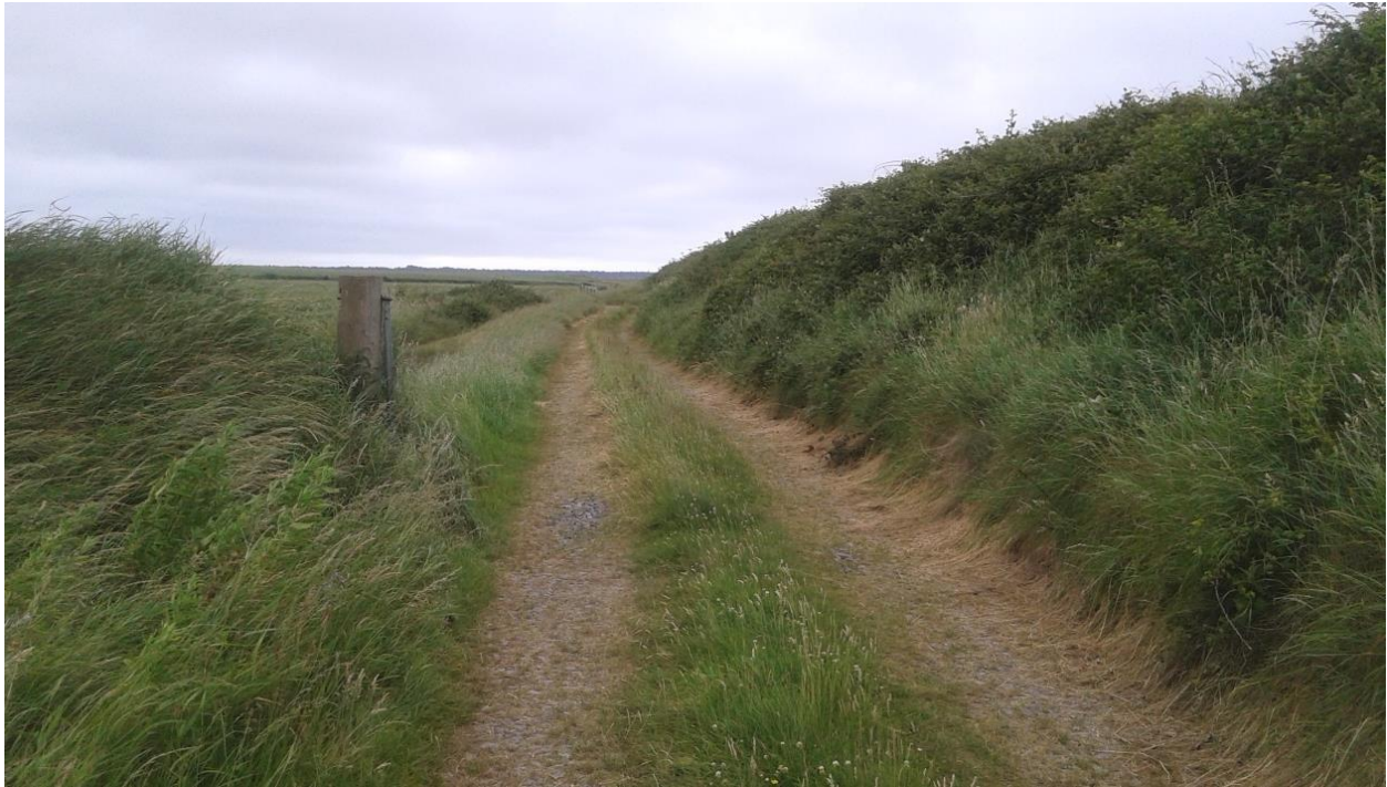
Fig. 4.10: Farm Lanes at Base of Sea Wall (Ch:4+000):
