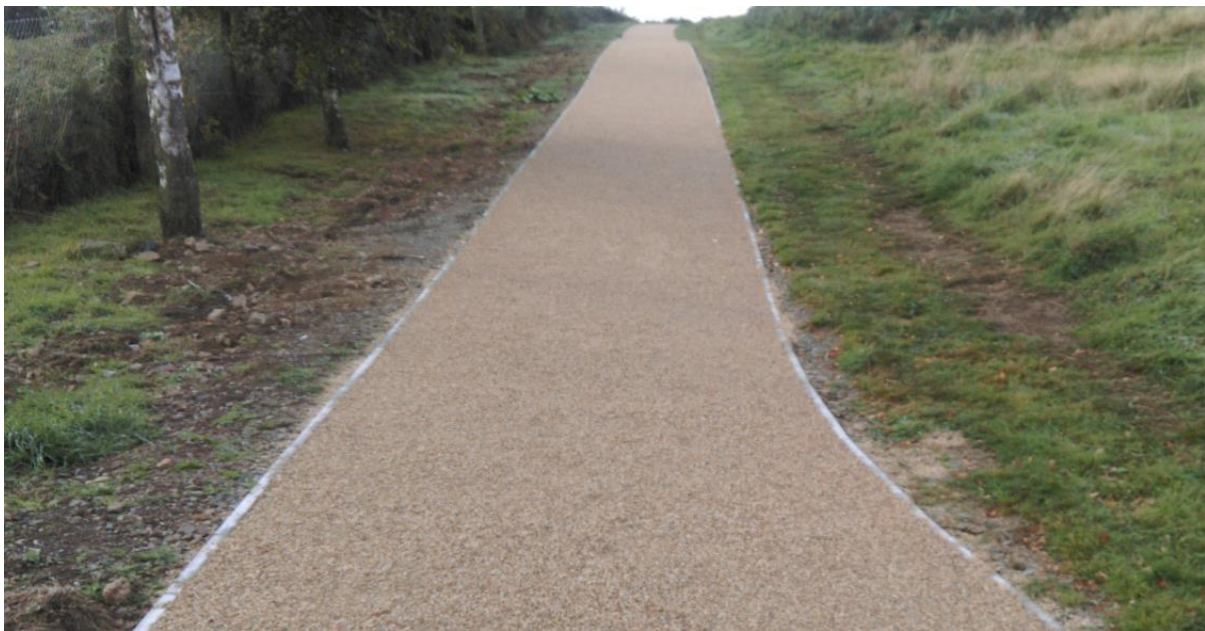
Fig. 7.3: Macadam Contained with Precast Concrete Edging:
