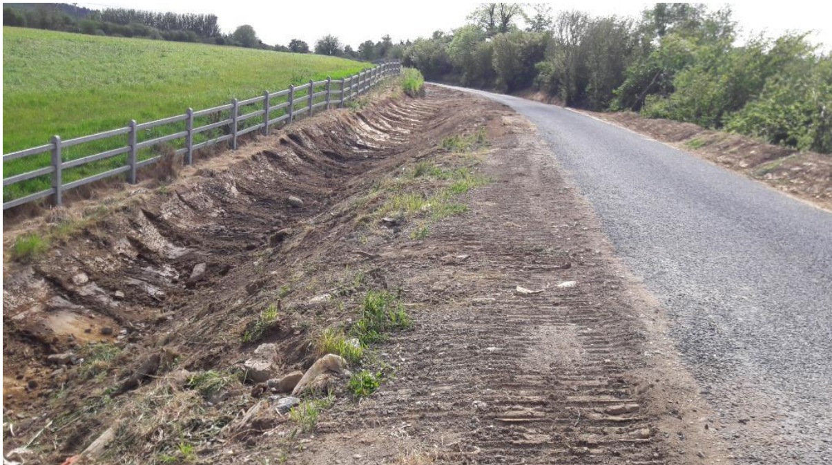
Fig. 7.9: Trail Runoff to Drainage Grip / Ditch:
