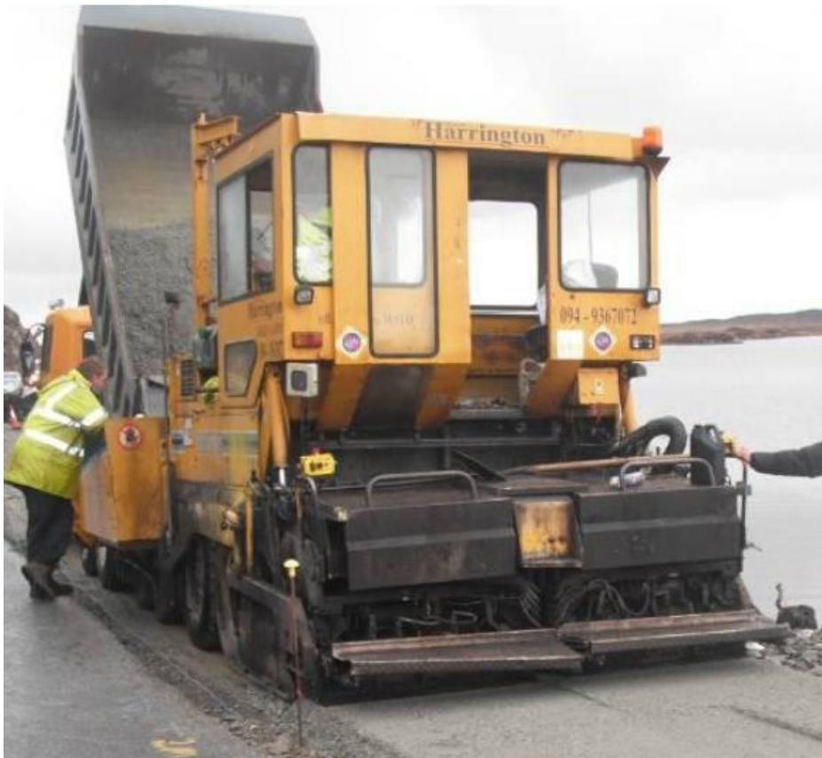
Fig. 7.1: Macadam Paving Machine Laying Sub-base:
