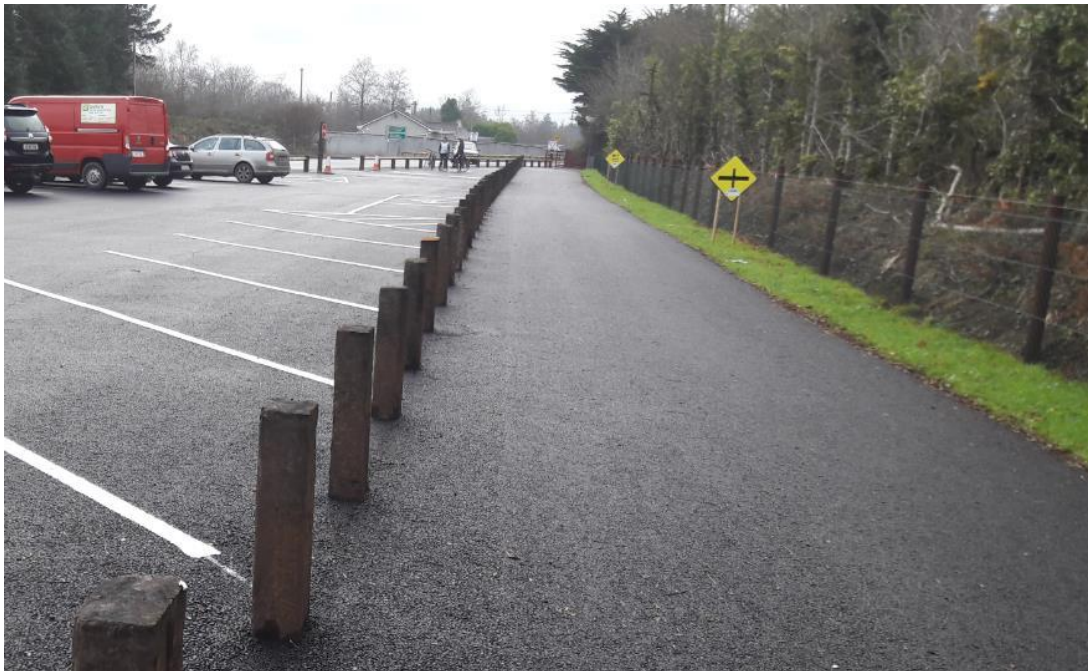
Photo B2: Bollards to restrict vehicles but not cyclists (Deise Greenway):
