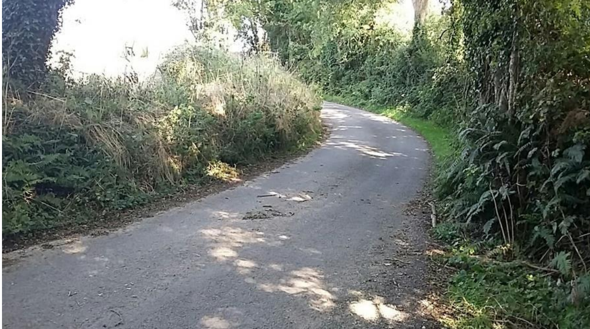
Fig. 3.4: Purple Route – Poor Visibility on County Road:
