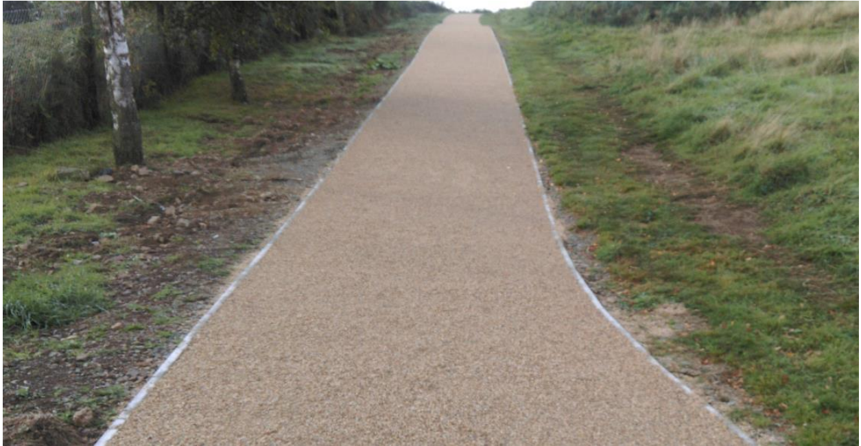
Fig. 2.1: Example of Typical Surfaced for a Greenway:
