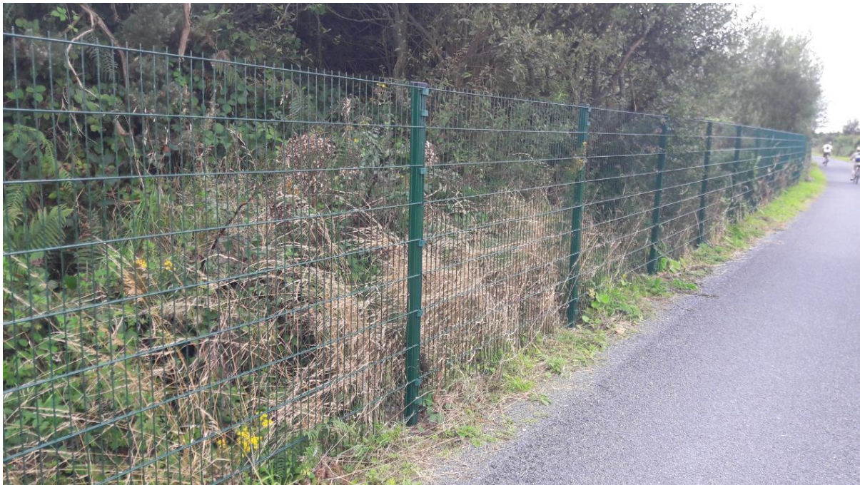
Fig. 7.11: 1.8m High Paladin Secure Fencing:
