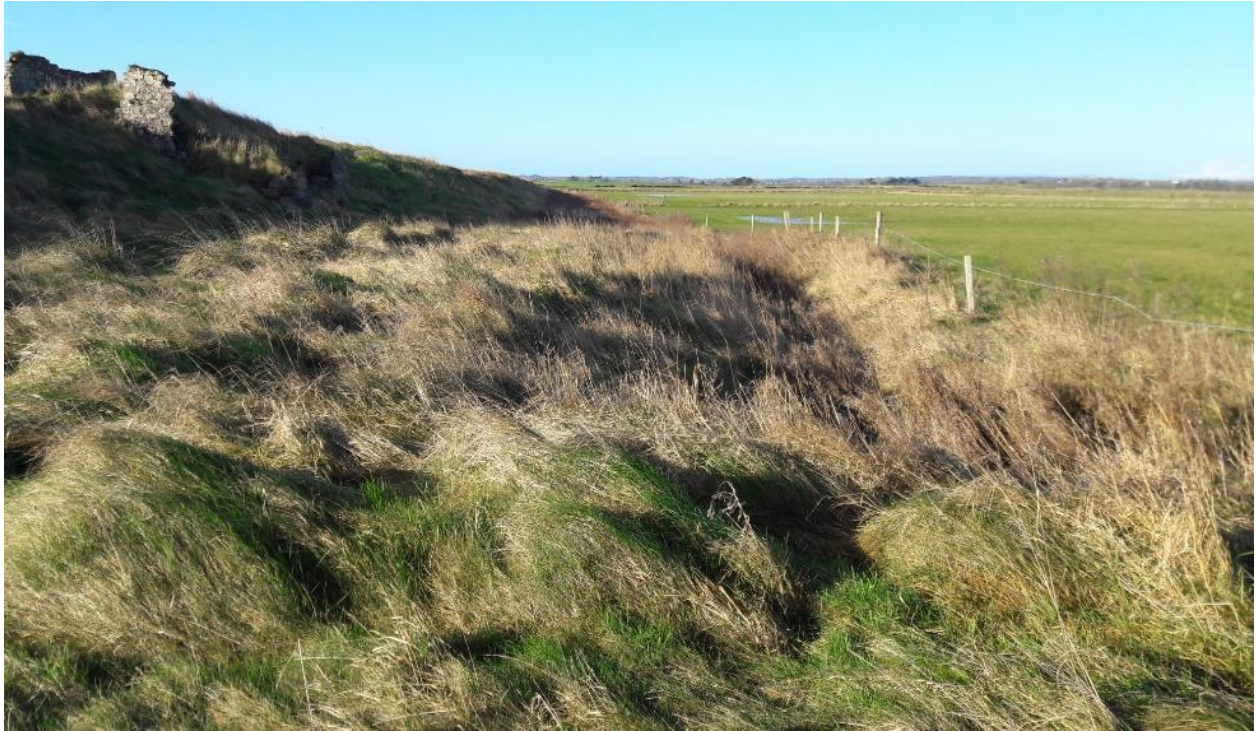
Fig. 4.3: Typical Yellow Route Corridor Along North Slob Sea Wall (Ch:6+000):
