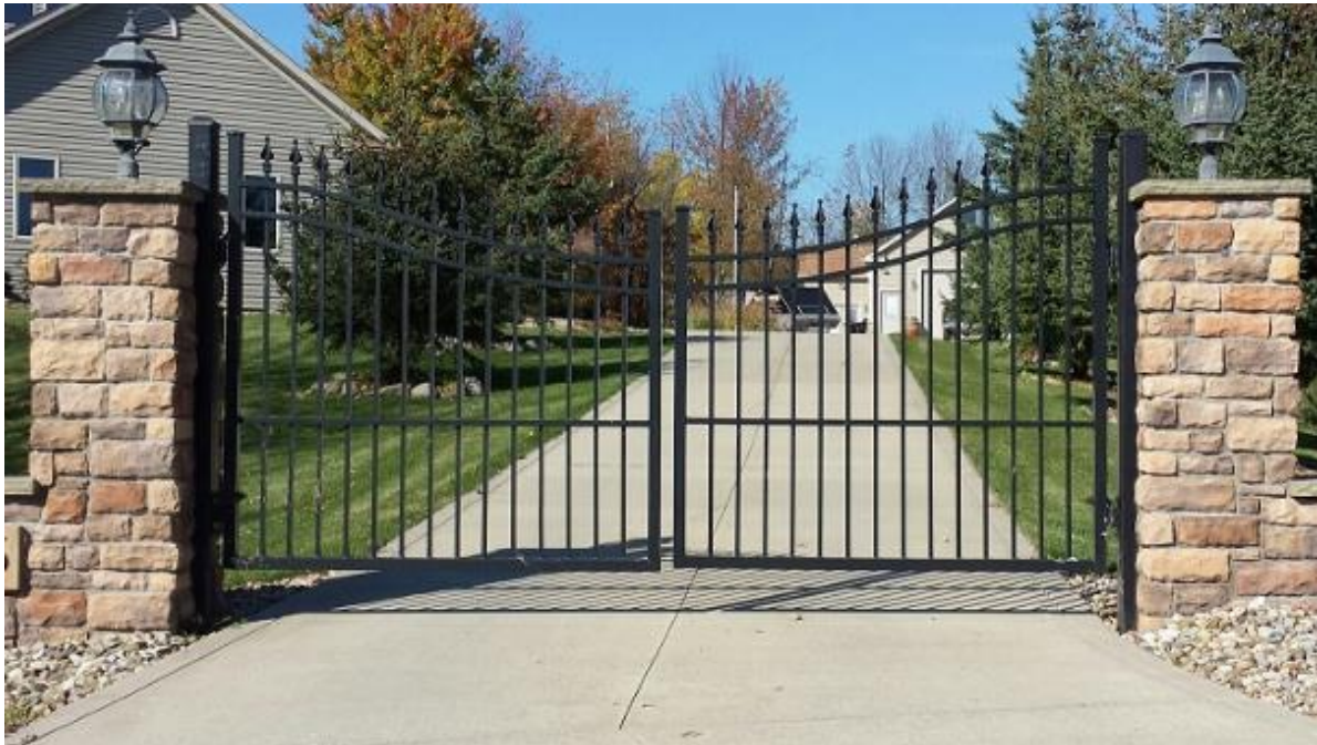
Fig. 7.12: Example of Secure Gate / Pier Combination:
