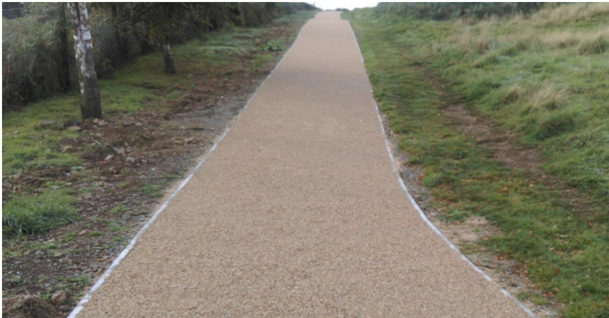
Fig. 3.2: Beige Coloured Macadam Contained by Precast Concrete Edging:
