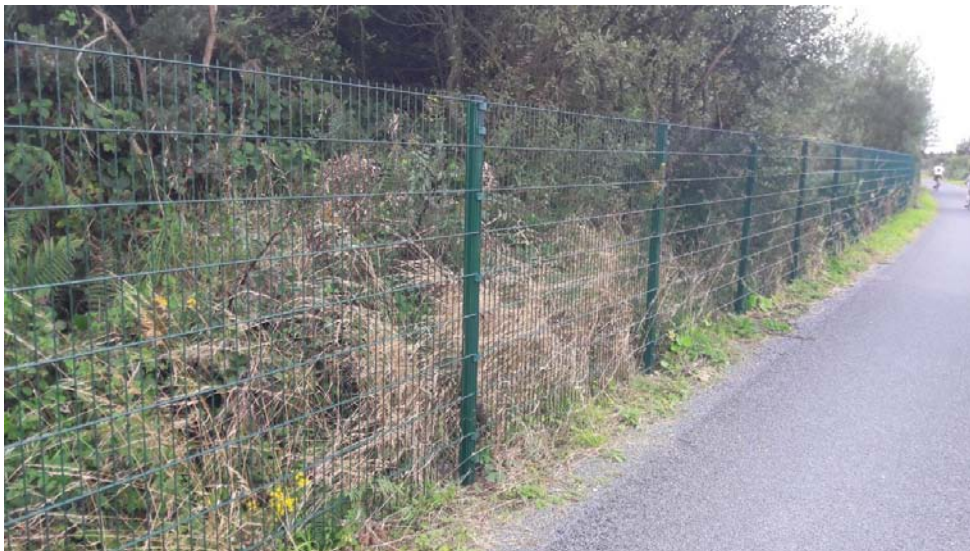
Fig. 3.5: 1.8m High Paladin Secure Fencing:
