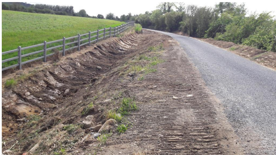
Fig. 3.7: Trail Runoff to Drainage Grip / Ditch:
