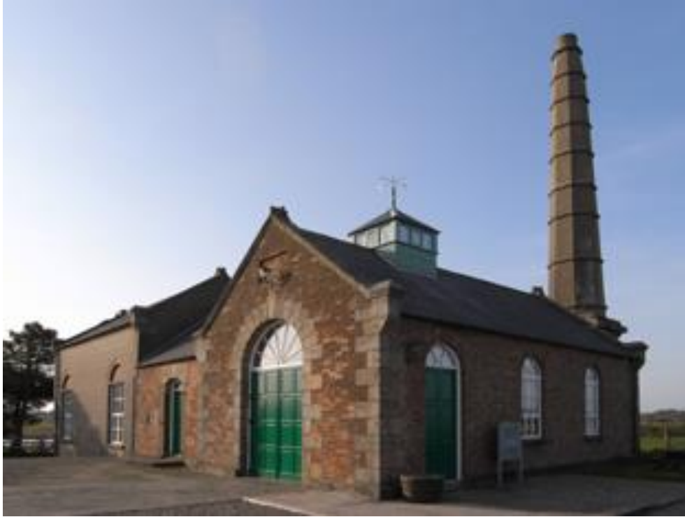
Fig. 5.7: North Slob Pump House (1845-1852) [NIAH 15703805]:
