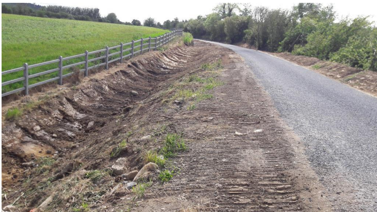
Figure 11: Greenway Runoff to Drainage Grip / Ditch
