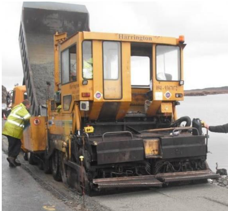
Figure 6: Macadam Paving Machine Laying Sub-base
