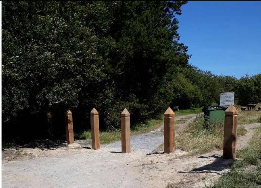
FIGURE NO.15 FENCING ERECTED AT CULLETONS GAP 2017
