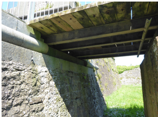
Fig. 126: Battered wall and bridge connection
