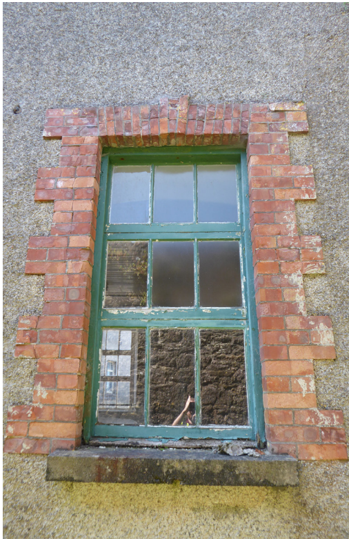
Fig. 81: Window to east elevation
