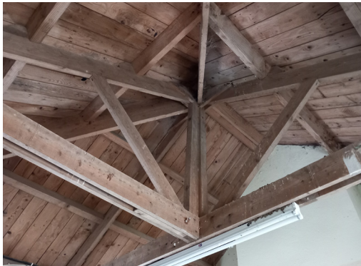
Fig. 75: Exposed timber truss roof structure
