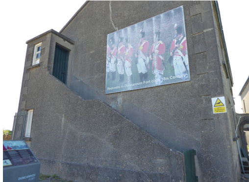
Fig. 63: East elevation with external stair to first floor
