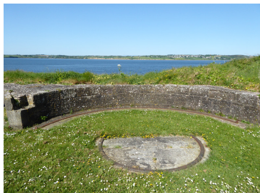
Fig. 15: North gun ring and central section
