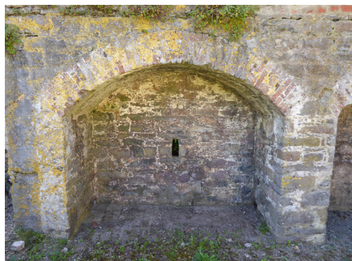
Fig. 123: Arch with central loop
