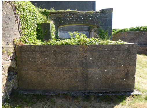
Fig. 66: West elevation, south side and bund
