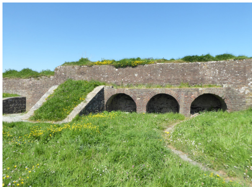
Fig. 120: Walls leading to southern turret
