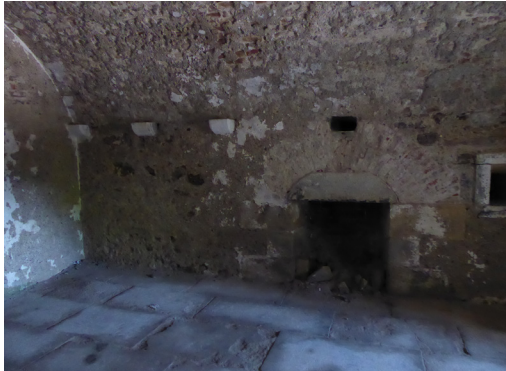
Fig. 130: Room five, fireplace
