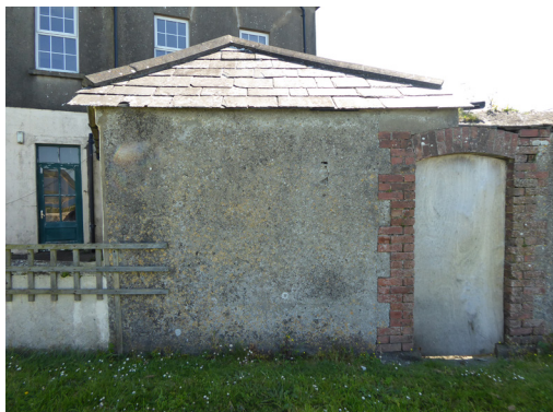
Fig. 56: Yard wall and return
