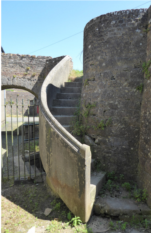
Fig. 98: Staircase to rampart
