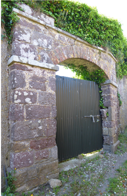
Fig. 96: Brick archway to rear yard
