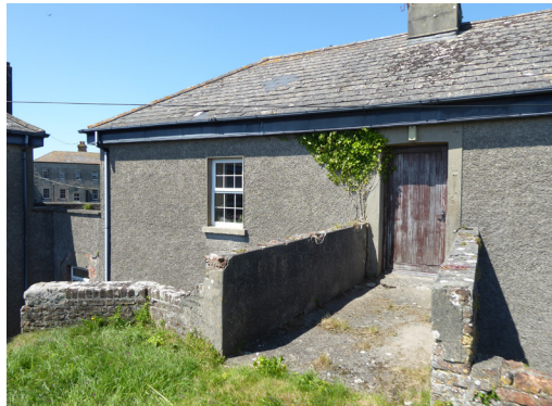
Fig. 83: First floor bridge to east elevation
