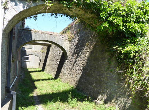
Fig. 97: Area south of bridge
