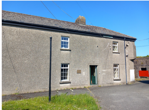
Fig. 87: South elevation, east side
