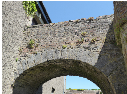
Fig. 84: Arch under bridge to east elevation
