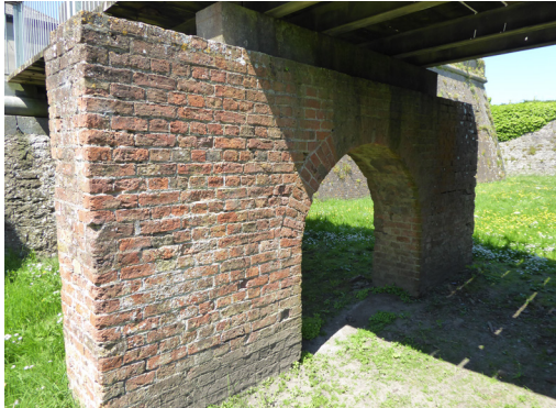
Fig. 125: Brick pier under bridge
