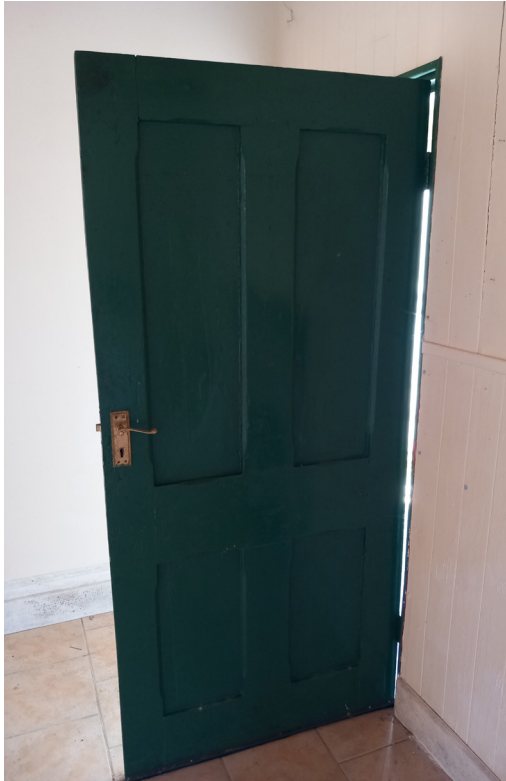
Fig. 86: Potentially original timber door
