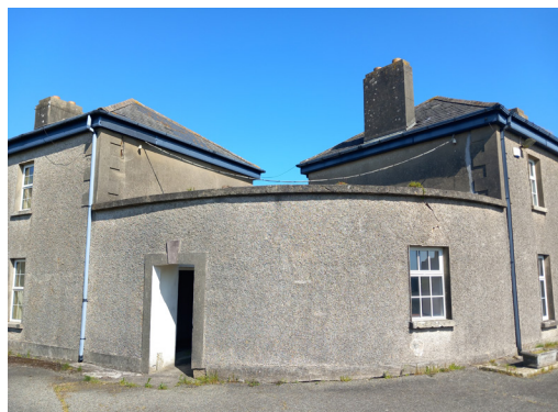
Fig. 79: Connecting wall between building No.10 &amp; 11
