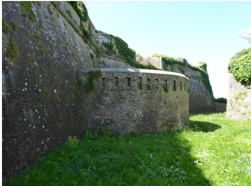
Fig. 113: Exterior wall, south side
