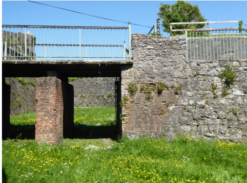
Fig. 102: East wall, north side
