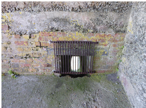
Fig. 27: Drainage chute to north wall
