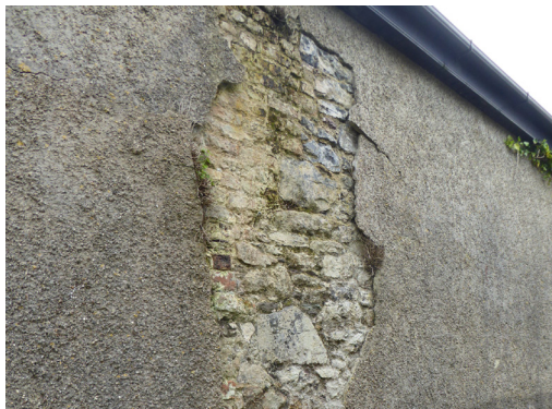
Fig. 45: Detached render to north elevation
