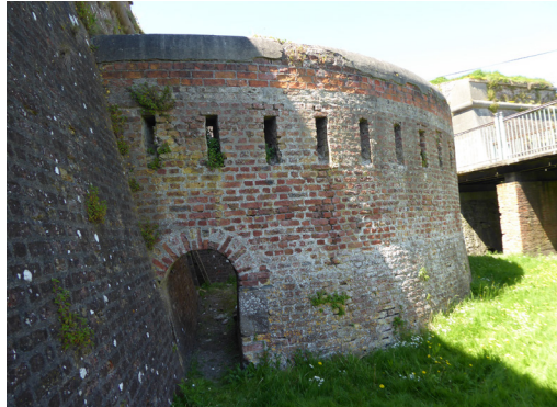
Fig. 111: Opening to interior
