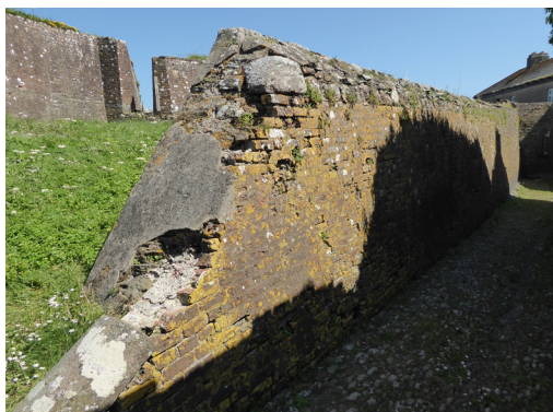
Fig. 101: Wall to northern passageway
