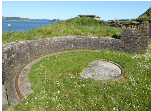
Fig. 14: North gun ring and wall to north
