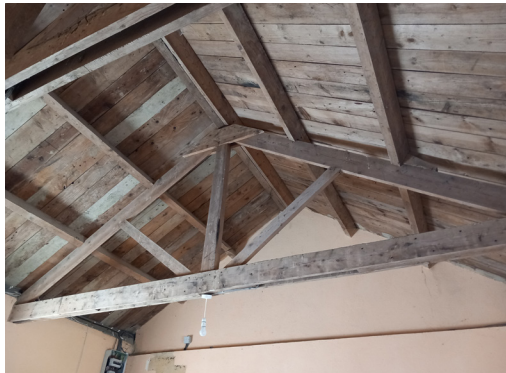
Fig. 92: Exposed timber truss roof structure
