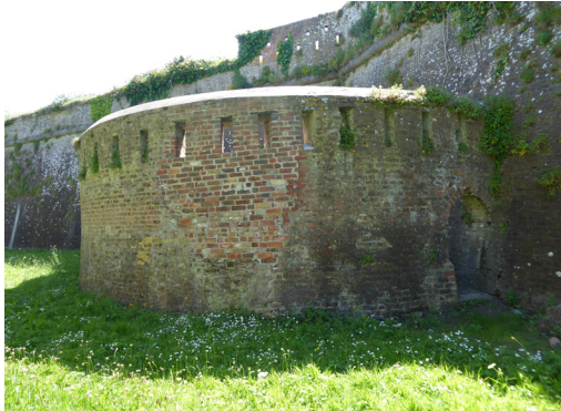
Fig. 114: Exterior wall, north side
