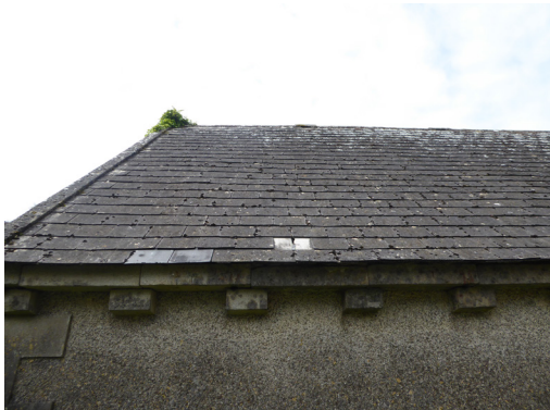
Fig. 31: Eaves course and corbels
