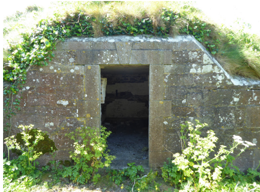
Fig. 16: Door opening to store
