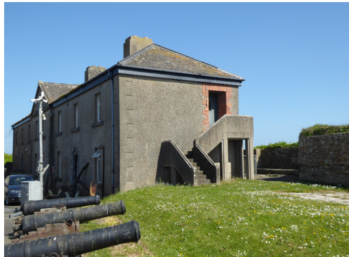
Fig. 72: West elevation with later stair to first floor
