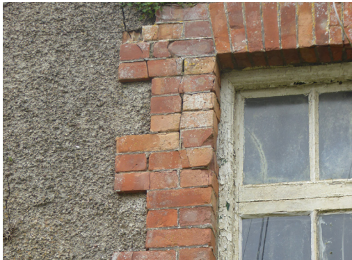
Fig. 44: Brick surround to east window
