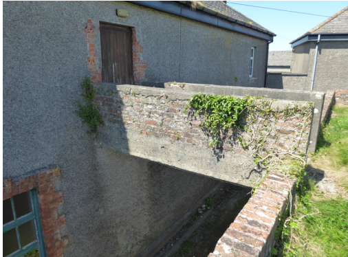
Fig. 80: First floor bridge to east elevation
