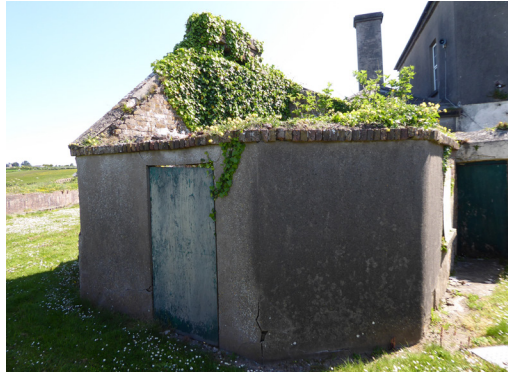
Fig. 69: West and south-west elevations
