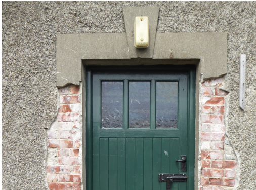
Fig. 43: Entrance door and surround
