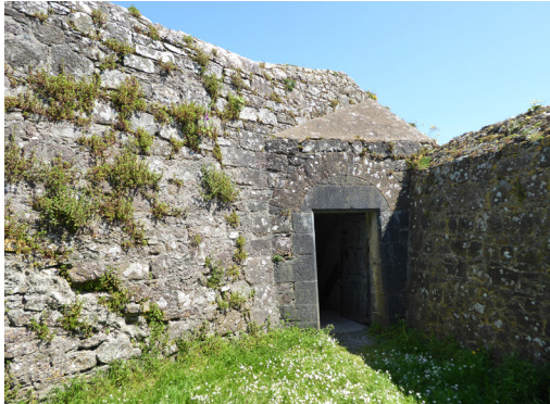
Fig. 103: East wall, south side
