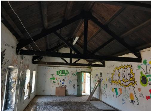
Fig. 95: Exposed timber truss roof structure
