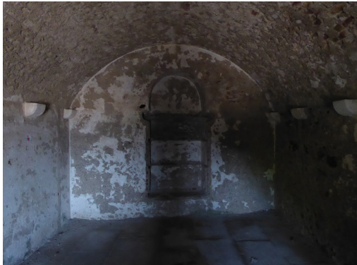
Fig. 129: Room five, recess
