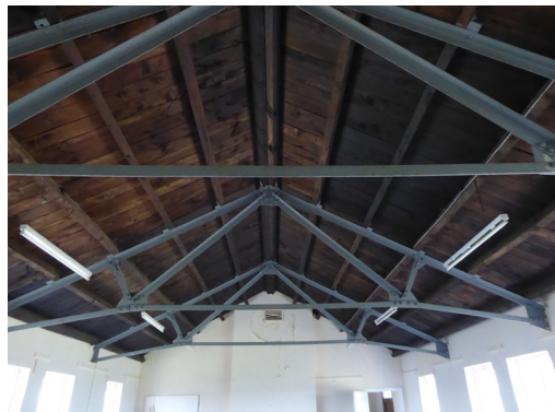
Fig. 48: Wrought-iron trusses
