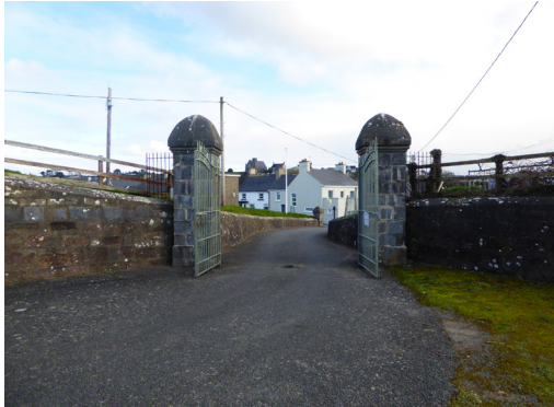
Fig. 133: Piers and gates leading to site
