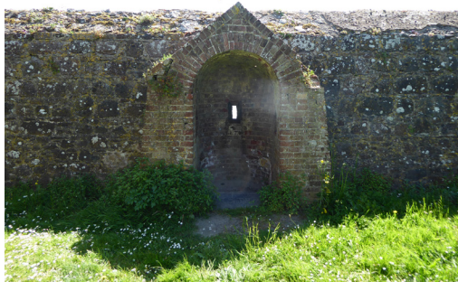
Fig. 104: Projecting gabled brick insertion in wall
