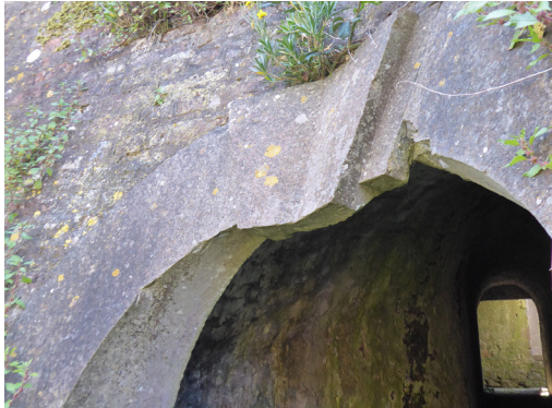
Fig. 107: Stone surround to tunnel entrance
