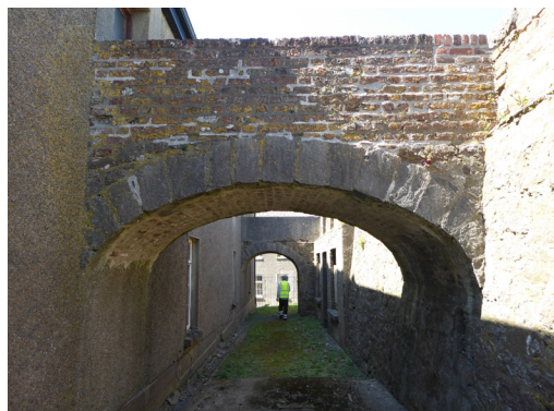
Fig. 89: Bridge archway, north elevation
